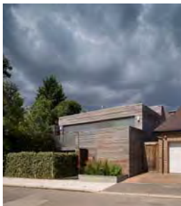
Figure 6-7. The occupants of the Passive House say south-facing blinds to the living spaces (that are all street-facing) are kept closed during the day in order to maintain privacy – they are kept closed during the winter months more than expected at the design stage. However tilting the blinds slightly upwards to allow sunlight to enter the house would solve the privacy concerns while also allowing the benefits of solar gain in winter.
