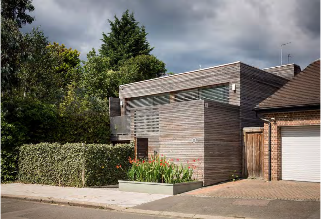
Figure 1-2b. South facing street elevation of the Camden Passive House, with living room on the first floor and bedrooms on the ground floor. Cladding is Austrian larch.
