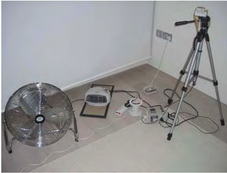
Figure 3-3. Camden Passive House: co-heating test equipment
