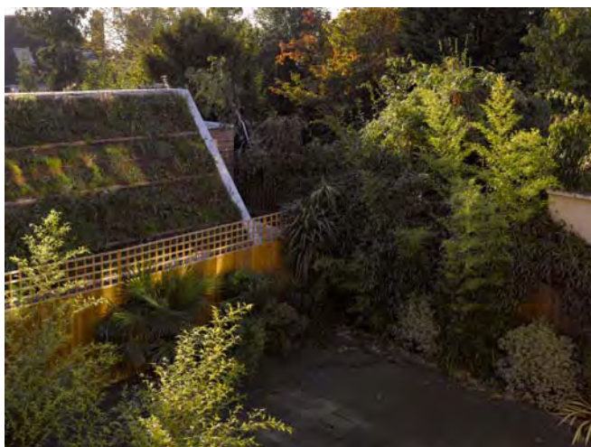
Figure 2-3. Sloping green roof facing neighbour's garden
